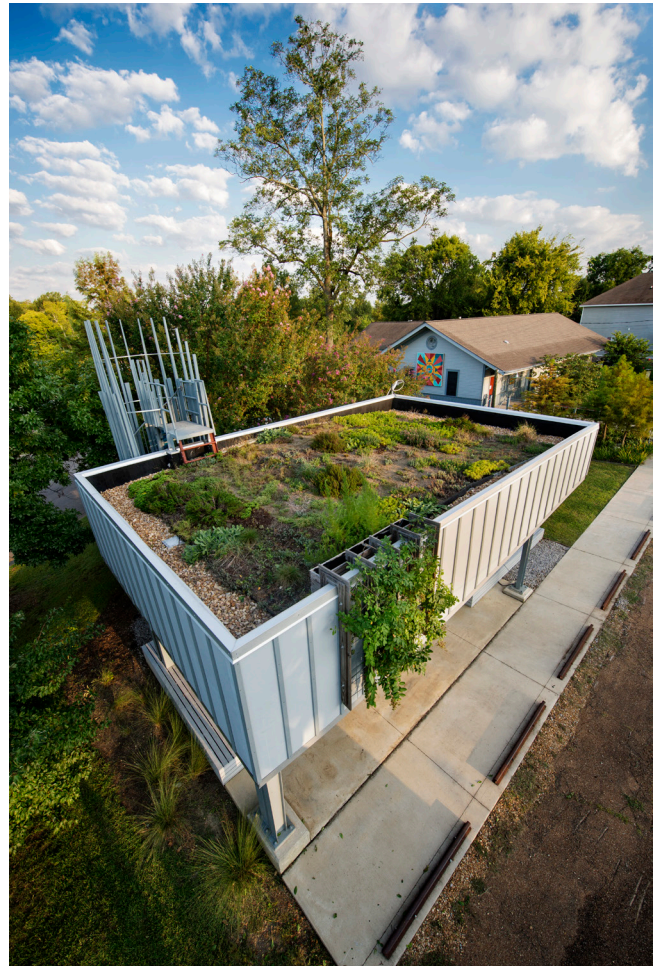
Figure 6. SuperUse Pavilion green roof and planted wall system hinting at what lies above.
