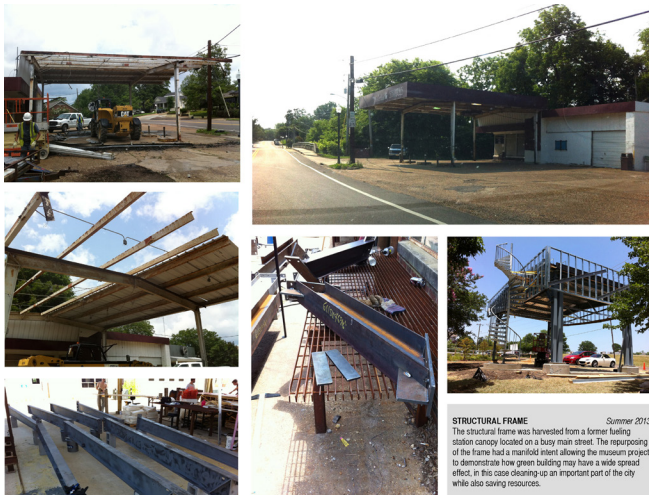
Figure 4. Former fuel canopy being dismantled, cleaned, reinforced, and erected.
